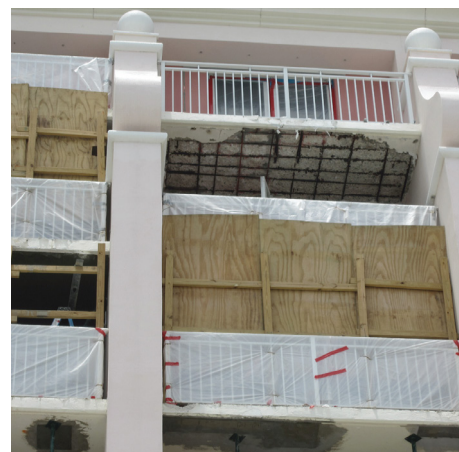
Plywood protection for rain water damage
